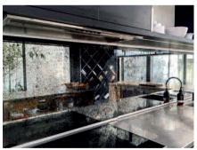
For those companies using a digital printer to create antique effects on glass, simply use our mirror spray and backing over the print to give unique reflective properties to the finished panel. (See right)
