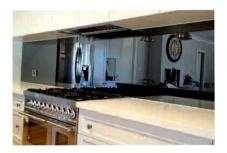
As mirror spray can go straight onto toughened glass, mirror finishes can now be used more widely in public areas which have strict health and safety guidelines on the thickness of glass used to restrict breakages.
